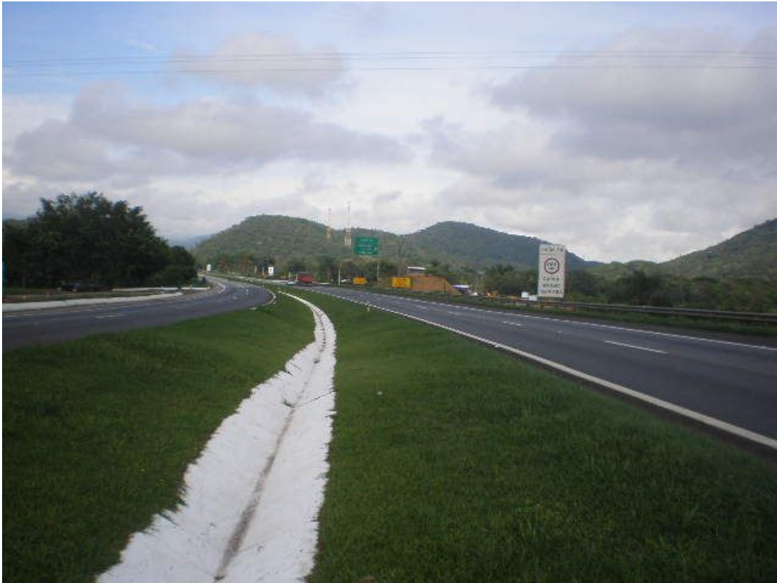
Figura 2.2 – Canteiro central, km 24,0 da BR-277/PR
